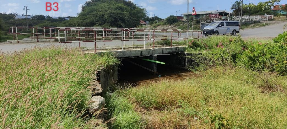
2=small maintenance should be done
