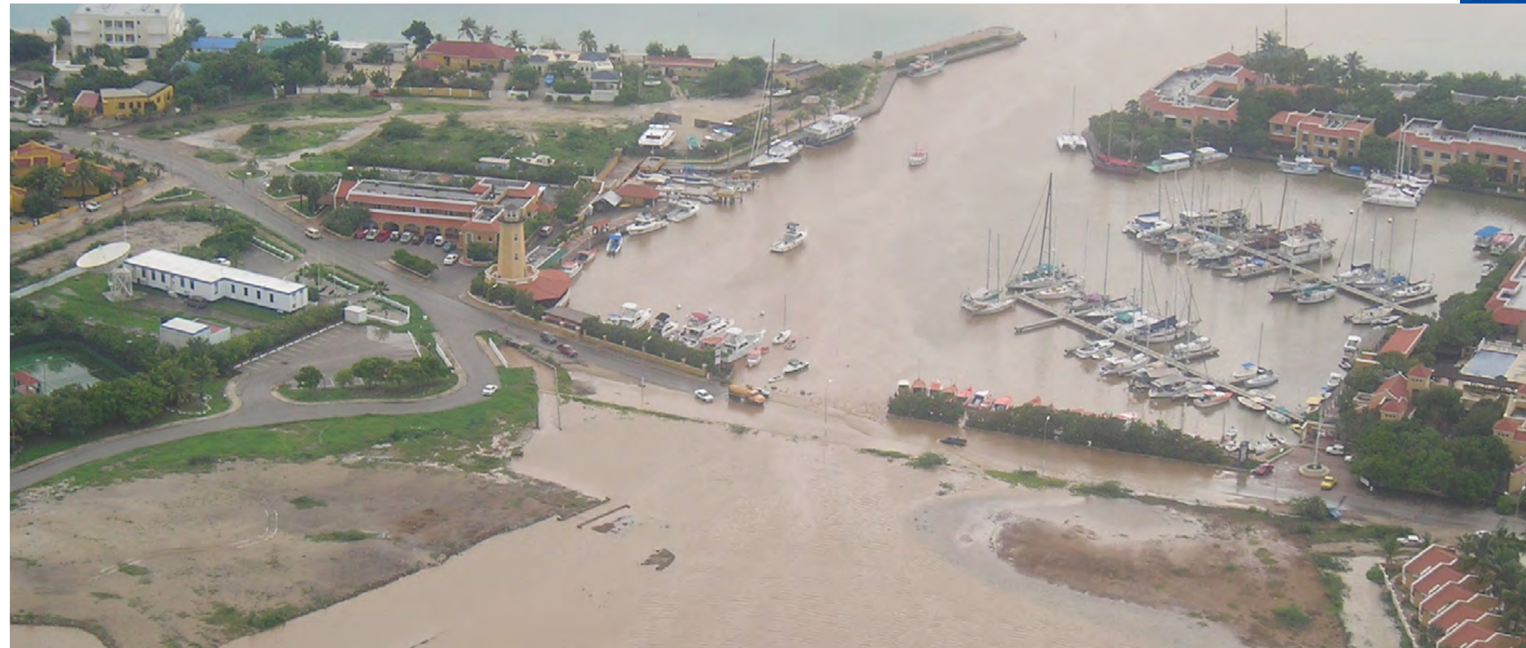
Overflow of Saliñas di Vlijt directly to the sea after heavy rainfall.
